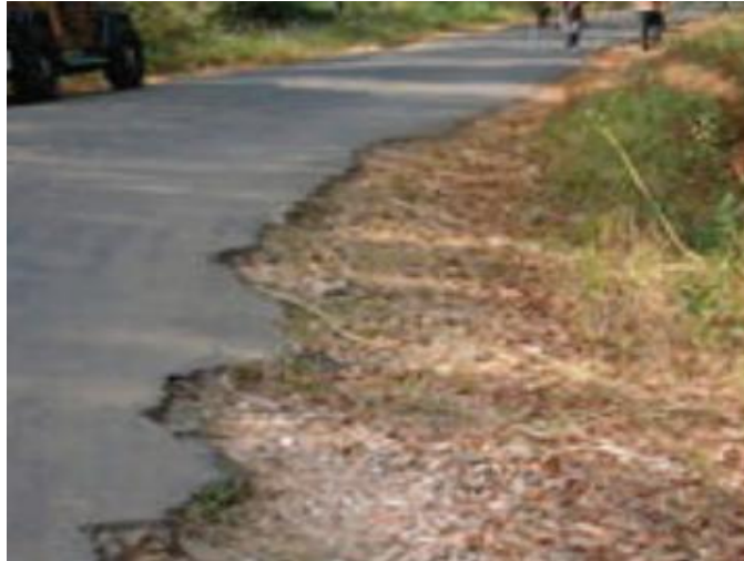
Figure 2.4: Damaged road edge
