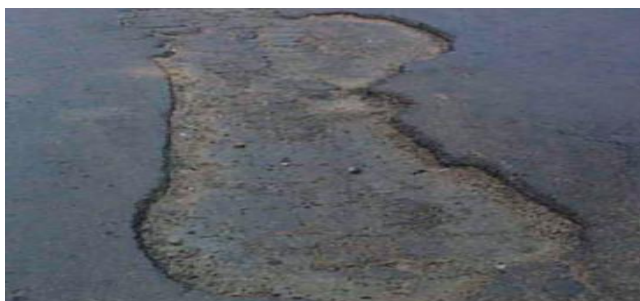
Figure 2.6: Delamination
